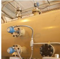
Improve tank operations and production separation through reliable, easy to use, virtually maintenance-free level and interface transmitters. Rosemount and Mobrey brand level products help manage your process and decrease the risk of spills that result in environmental damage.
