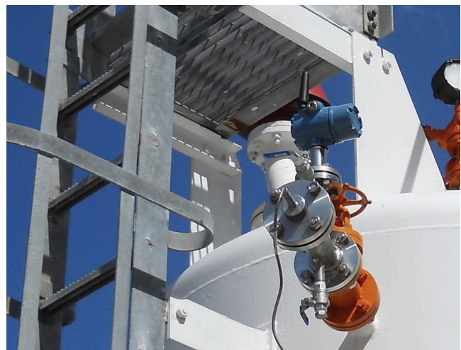
Rosemount 2160 installation
