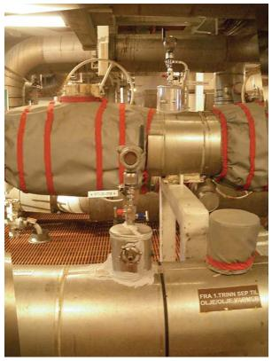
The Rosemount Smart Wireless pressure transmitters are used to measure pressure drop over the platform heat exchangers.
