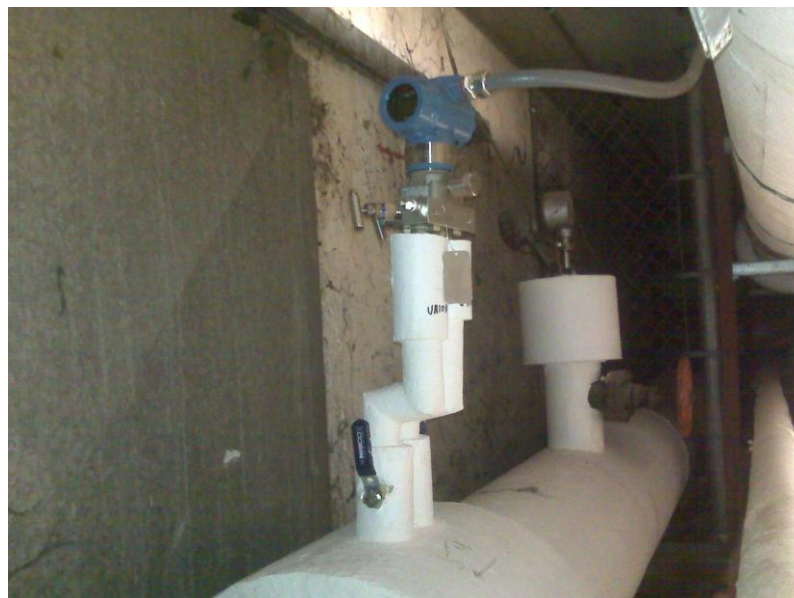
Figure 8: Remote mount transmitter, mounted above the pipe.
