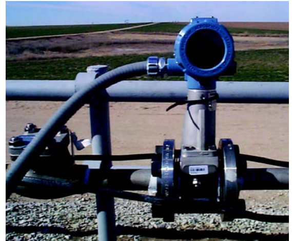
The Rosemount 8800 vortex flowmeter
