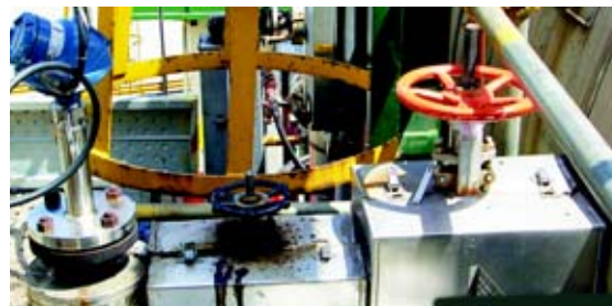
Rosemount Guided Wave Radar site installation
