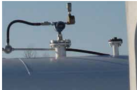
Figure 1. Installed Rosemount Smart Wireless THUM Adapter
