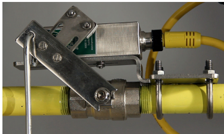
Figure 25: Safety Shower Valve in Activated Position
