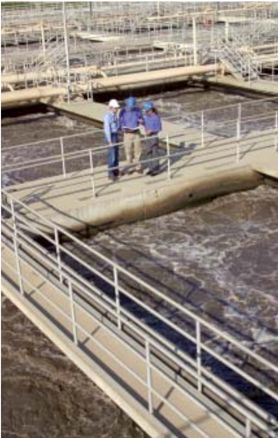
Aeration basins benefit from proper control of dissolved oxygen.
