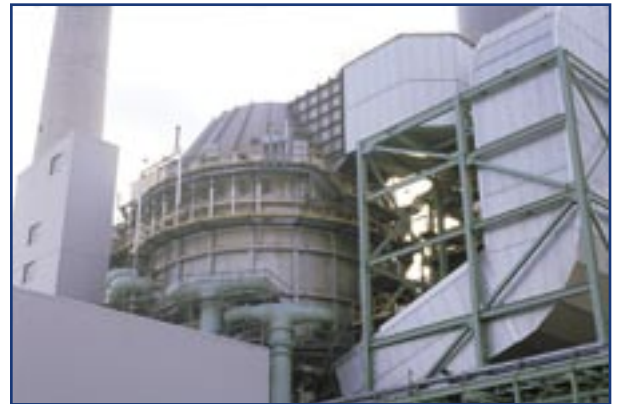
Use of technologies like a flue gas desulphurization system helps to secure Yonghung's place as one of the most clean and efficient power plants in the world.
