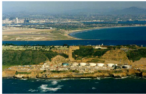
The Point Loma Water Treatment Plant is one of three new facilities constructed for the San Diego COMNET Project.
