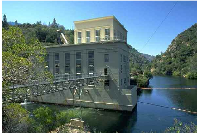
Big Creek Power House #8
