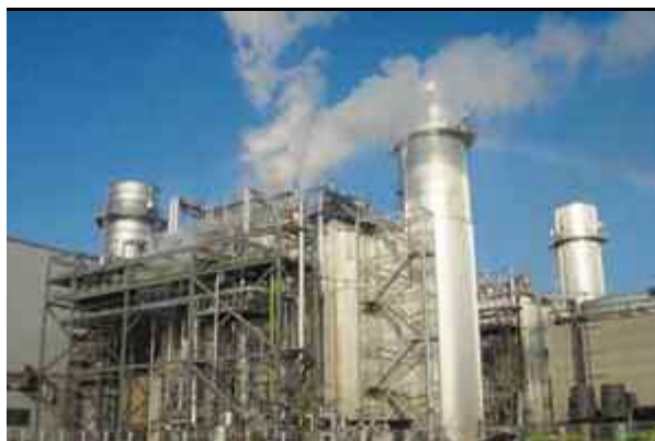
RATCHABURI POWER COMPANY LIMITED Ratchaburi Combined Cycle Power Plant Located in Ratchaburi, Thailand
