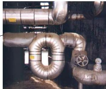
*CMF400 enclosed in an insulated heat jacket*
