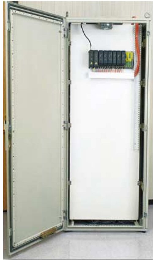
Figure 4. DeltaV with FOUNDATION fieldbus required panel space
