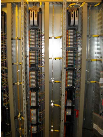
DeltaV Version 11 System Installed at the Plastics Lab
