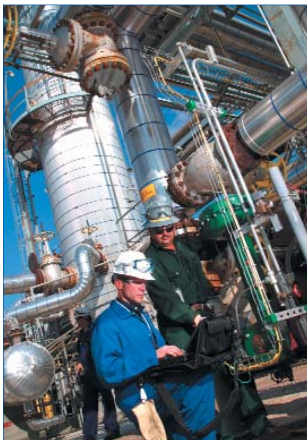
Figure 6. Emerson's ValveLink software gives full valve and positioner information during hot cutover.
