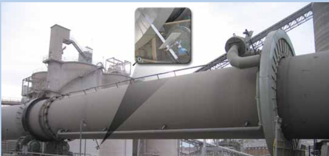
CalPortland's innovative application of wireless to monitor temperature distribution in a rotating kiln 540-ft. in length helped the company meet nitrogen-oxide emissions regulations and bag the top prize in Emerson's Smart Wireless Innovators contest this year.
