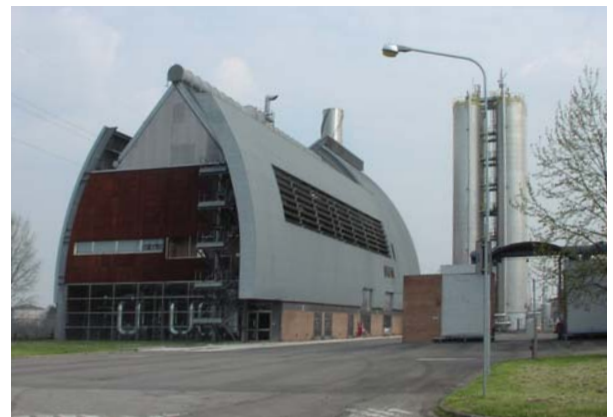
Reggio Emilia Cogeneration Site.
