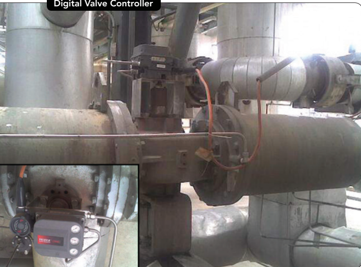
Figure 1. Unit features reliable and accurate linkage-less, non-contact valve-stem feedback technology.
