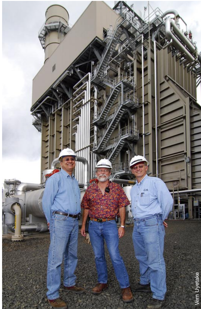
3. Balance-of-plant critical loops are controlled via the digital bus—including the HRSG’s drum-level signal and feedwater flow. From left in front of boiler are Jaisen Mody, engineering/construction/startup manager; Mike Schwartz, plant manager; and Bill Monroe, plant engineer
