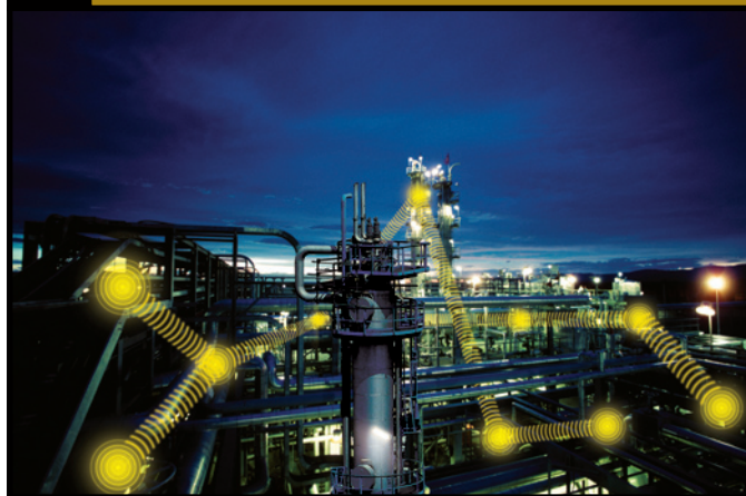
Figure 3. Signals are automatically routed around any blockages, and new devices automatically connect up.
