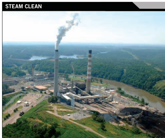
Alabama Power's Gorgas Steam Plant uses an in-house oil analysis system to avoid catastrophic events by checking machinery health.
